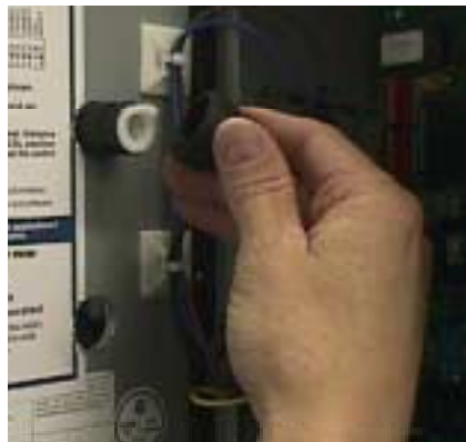
5. Install operator in hole labeled PROGRAM 1-2-3 . Re-install and tighten the locking nut and relatch the contact block assembly.
