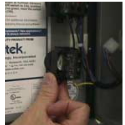
6. Repeat process with momentary contact operator. Mount in hole labeled RESET .
