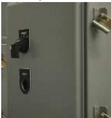
4. Loosen and remove the bayonet locking nut.
