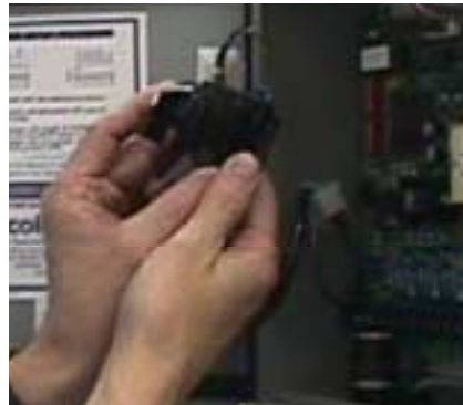
2. Unlatch contact block from rear of 3-position switch.
